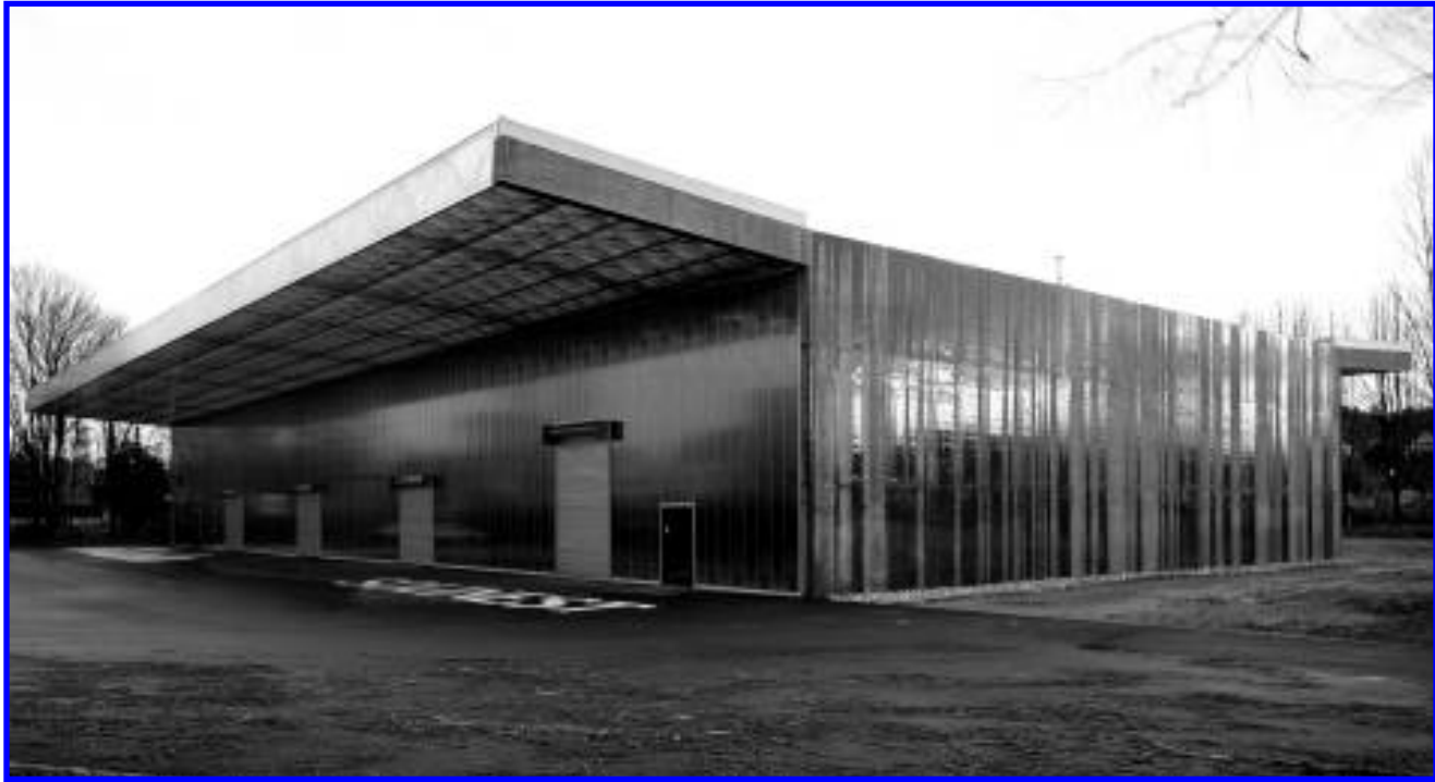
Fig. 2. Herzog & de Meuron Architects, Ricola-Europe SA Production & Storage Building, Mulhouse-Brunstatt, France (1993). (Photo © Margherita Spiluttini) The structure is designed to drain rainwater onto a vertical wall surface. When sunlight interacts with environmental conditions, it creates a constantly changing surface reflection, which challenges the building's materiality.
